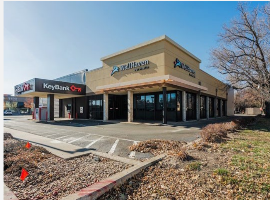
2305 S Colorado Blvd, Denver, CO
